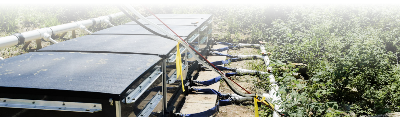
Figure 4. CAPTURE™ installation with boxes in parallel for runoff and tile treatment of 100 acres. (See site installation information at: https://youtu.be/POPVedDvZg8?si=EO4diP9Qpyie5a3e&t=127 .)
